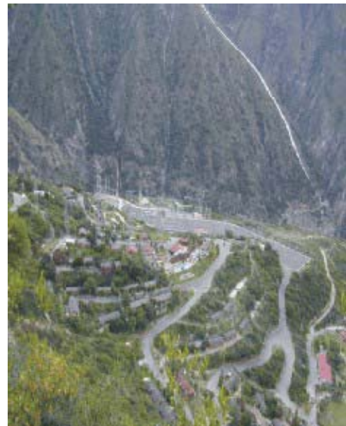
Figure 05: Partial view of the Mantaro Hydroenergetic Complex
