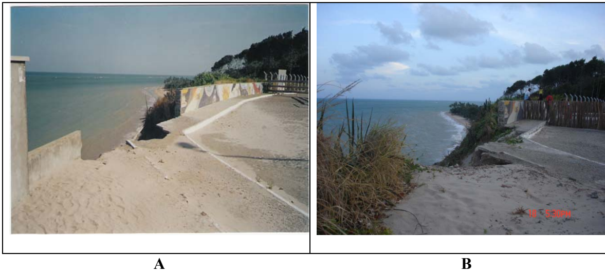
Figure 2 - Destruction of the “mirante” of the “Farol do Cabo Branco” at “Ponta do Seixas”, more eastern point of Americas, in João Pessoa - PB. Left picture (A) was taken on 2005 January and right one (B) on 2006 January. We can see the increasing destruction of the wall where the people using to see the sea.
