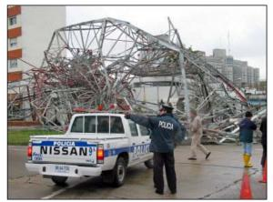
Figure 1 FM radio tower turn upside down in Montevideo, due the high winds during the 23-24 August 2005 event.
