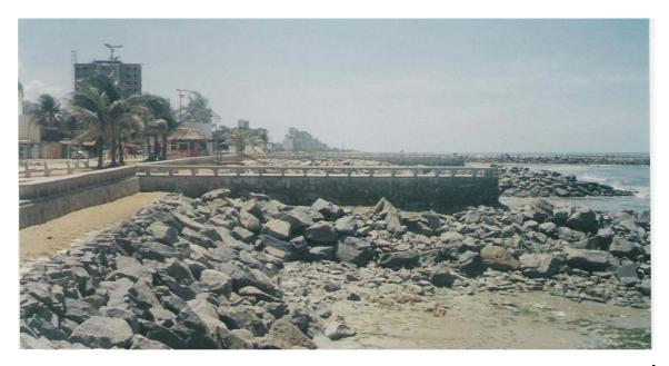
Figure 4 - Edge of Olinda, "Senator Marcos Freire" Avenue, where if they can notice the workmanships of containment of the advance of the sea where long ago the Bar's existed that had been transferred to the left side of the avenue.
